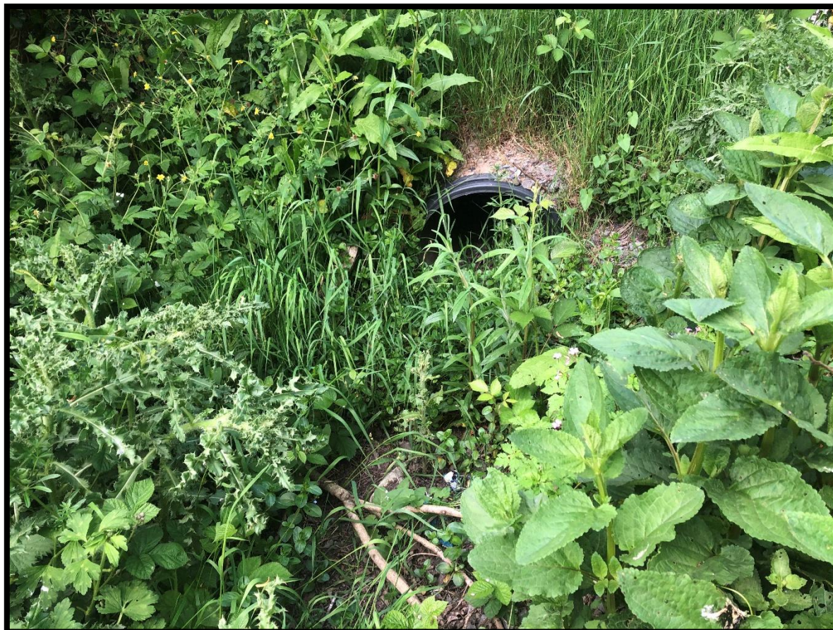
Plate 6.10 Image of a drain adjacent to the stream to the west
